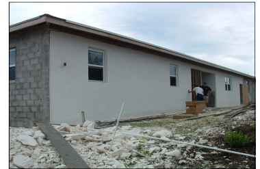
Significant progress on the mission house up on the hill.
